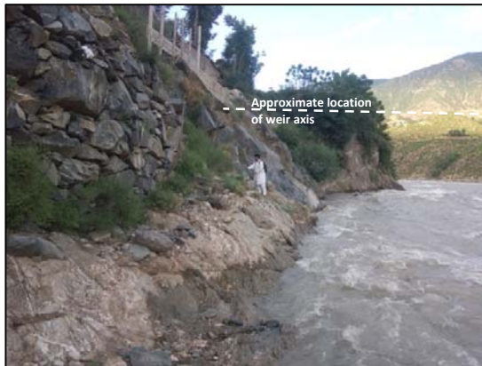
Figure 5.14: View of the left abutment where rock is present.
