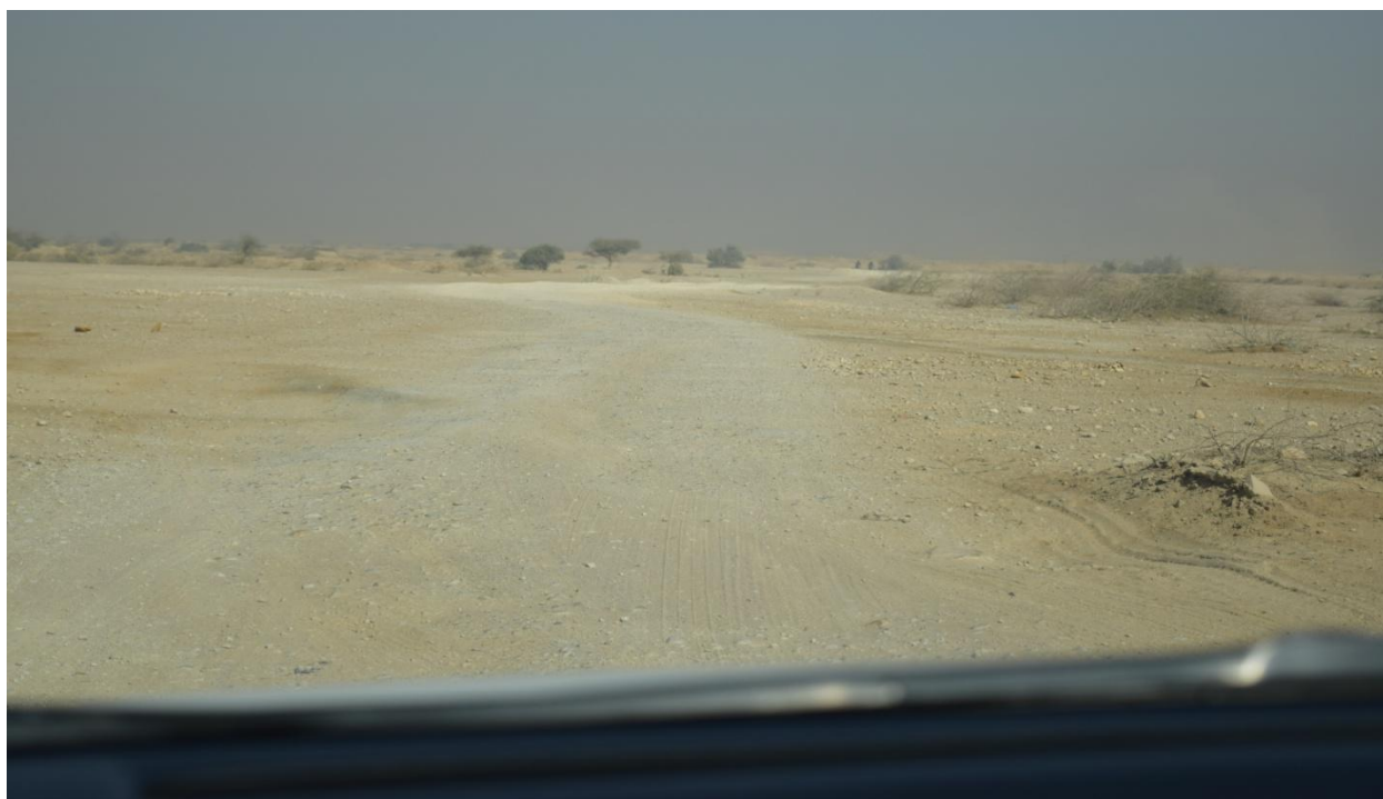
Figure 3.7: Unpaved Road towards Project Site
