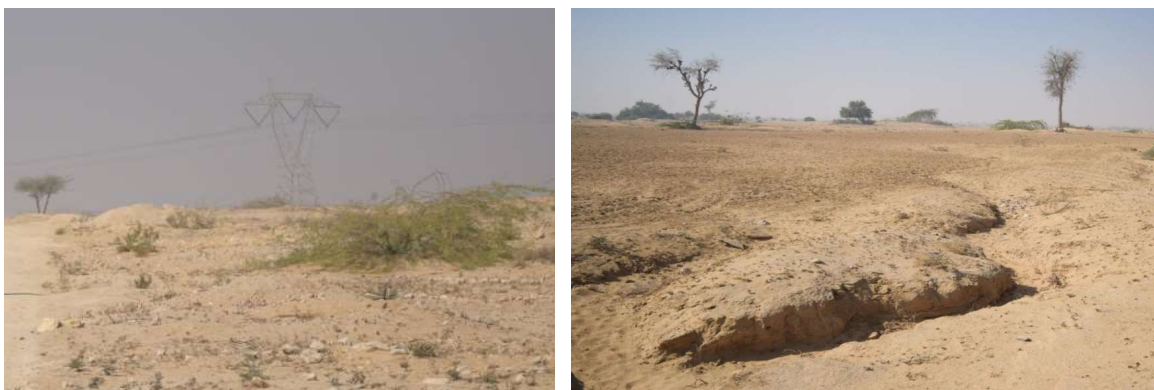
Figure 30 showing the 500KV pylon and trees that can cause shading
