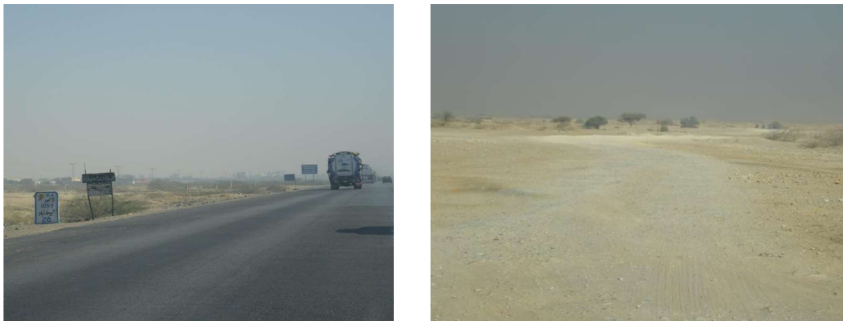
Fig 29 showing the existing M9 motorway and access road to the site.
