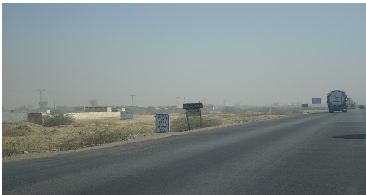
Figure 3.6: Karachi-Hyderabad Motorway –Road Overview
