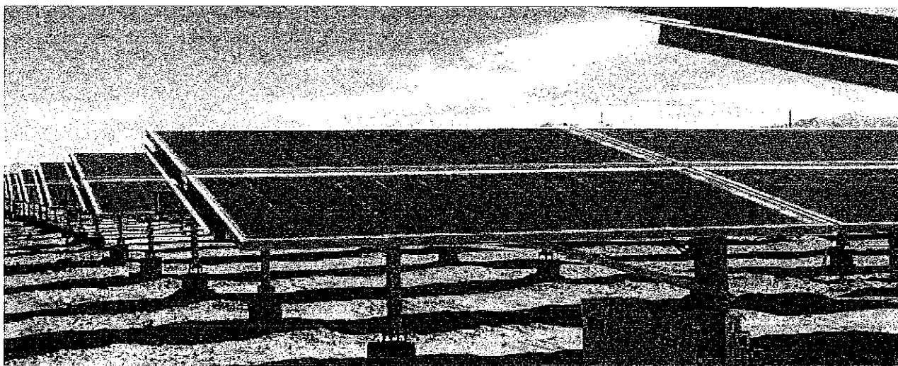
Figure 14 The horizontal single axis tracker
