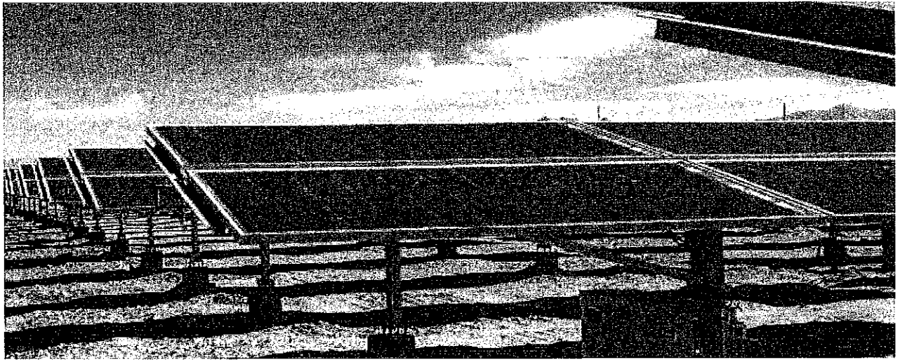
Figure 14 The horizontal single axis tracker
