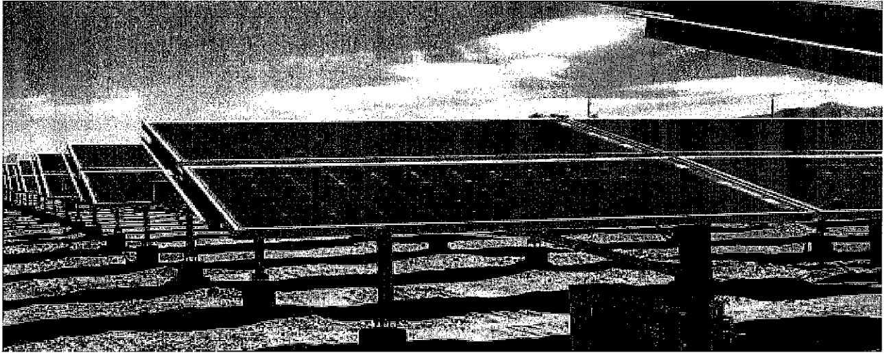
Figure 14 The horizontal single axis tracker
