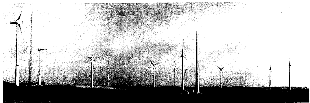
Figure 2.13 showing 11 x 7,5 MW E126 Estinnes Windfarm, Belgium, July 2010, one month before completion, with unique 2 part blades.
