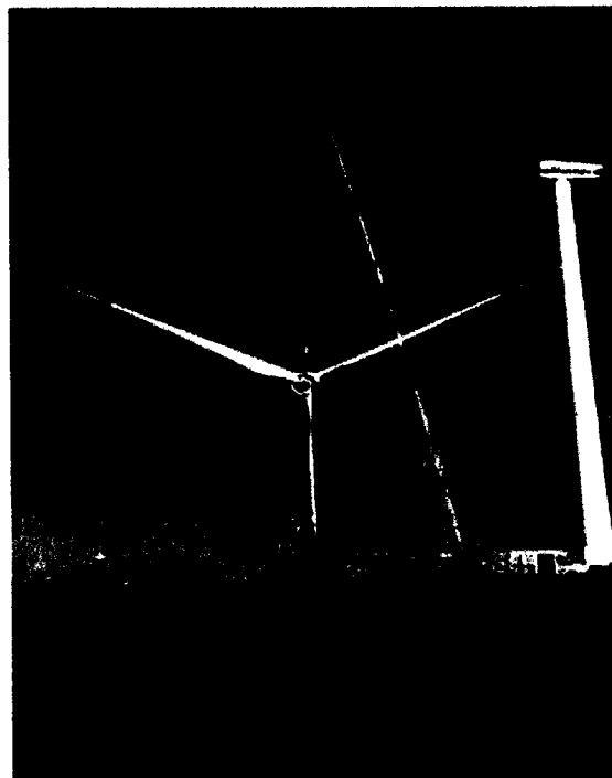
Figure 2.12: Installation of Nacelle and Blades
