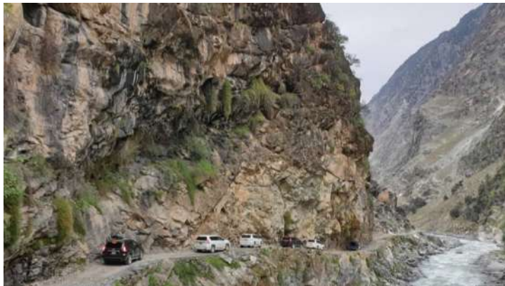
Section 2: narrow road section with overhanging rock slopes
