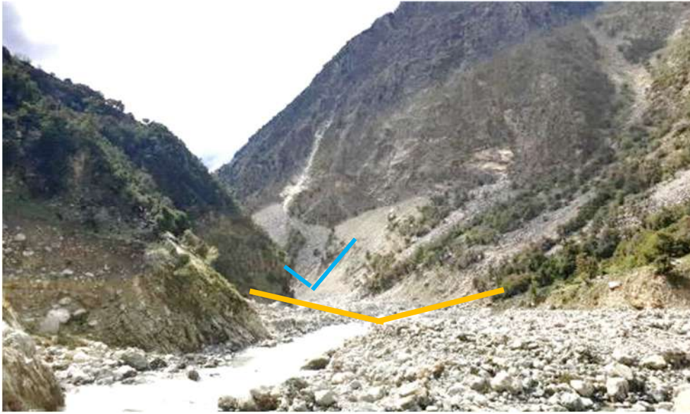
Figure 6-3: Dam site (blue: axis 2010; brown: weir axis 2020-2021) (view towards downstream)
