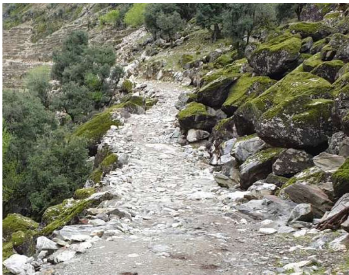
Section 4: alternate road surface (gravel and rock surface)
