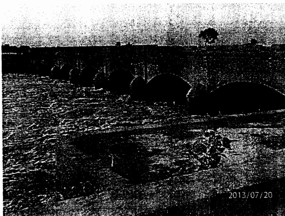
Figure 3.3: Fall Structure at RD 285+454
